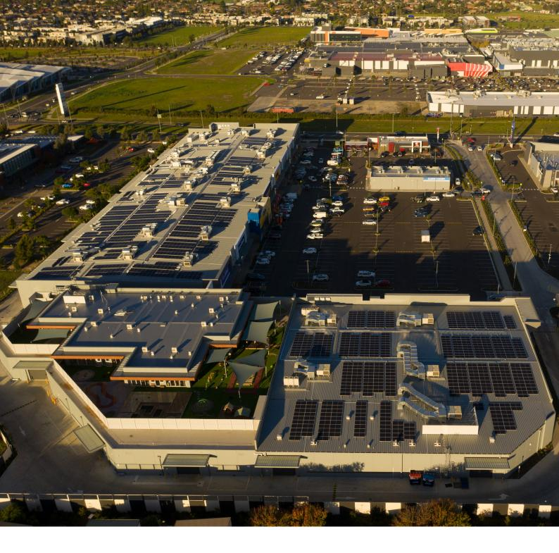
1MW solar PV system generating 1,332MWh annually
